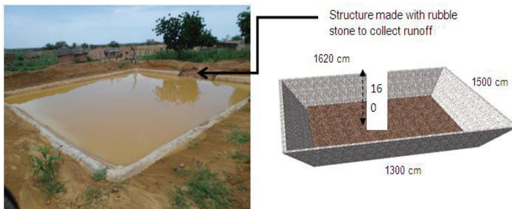
Figure 4. View of the studied rainwater harvesting basin (left) and its dimensions (right).
